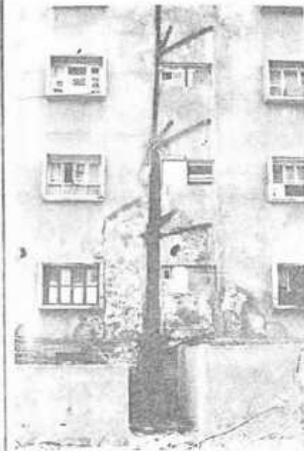
Plate 5 Vertical Cracks
