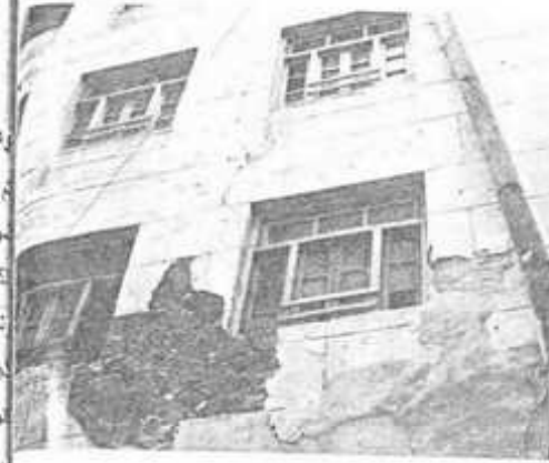
Plate 9 Diagonal Cracks
